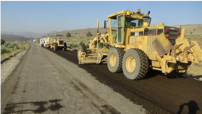
Grading and compaction
