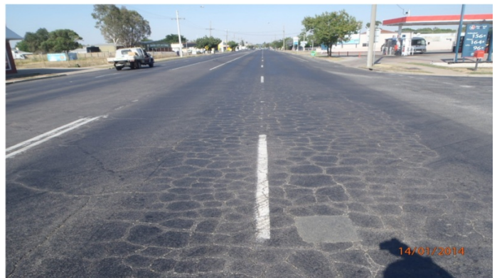
Pre-existing Condition - January 2014
