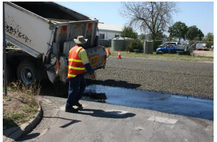
Installing the seal February 2014
