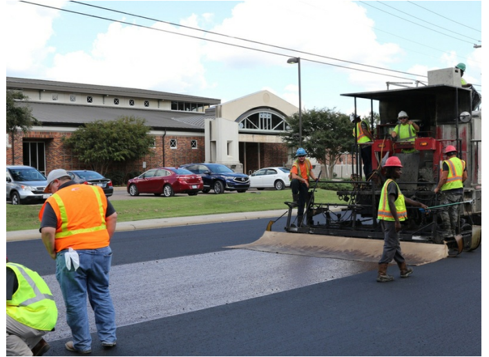
Scrub seal and premium micro surfacing was applied to this high traffic road in Rankin County.
