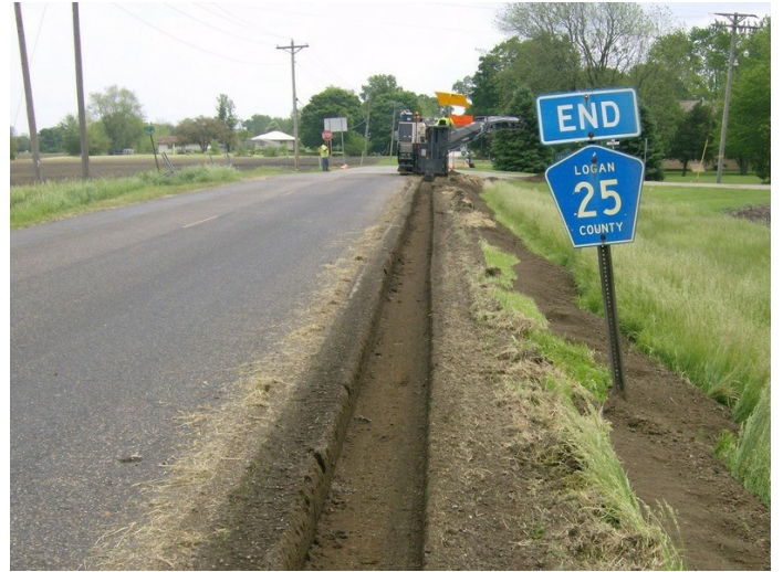
Trenching Material for Wideneing with FDR
