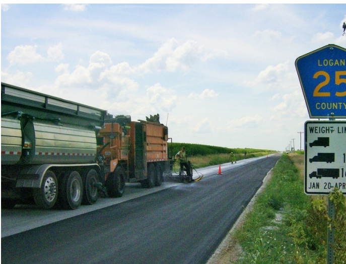
Applying the Microsurfacing
