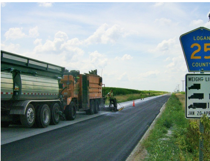
Applying the Microsurfacing
