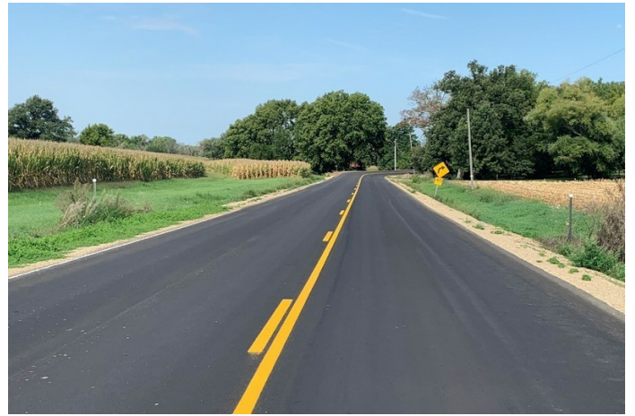
Finished Project with Cape Seal Surface
