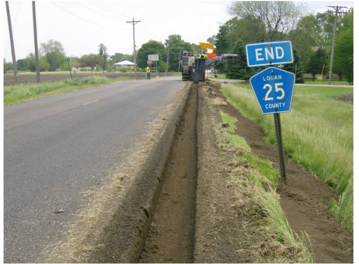
Trenching Material for Widening with FDR
