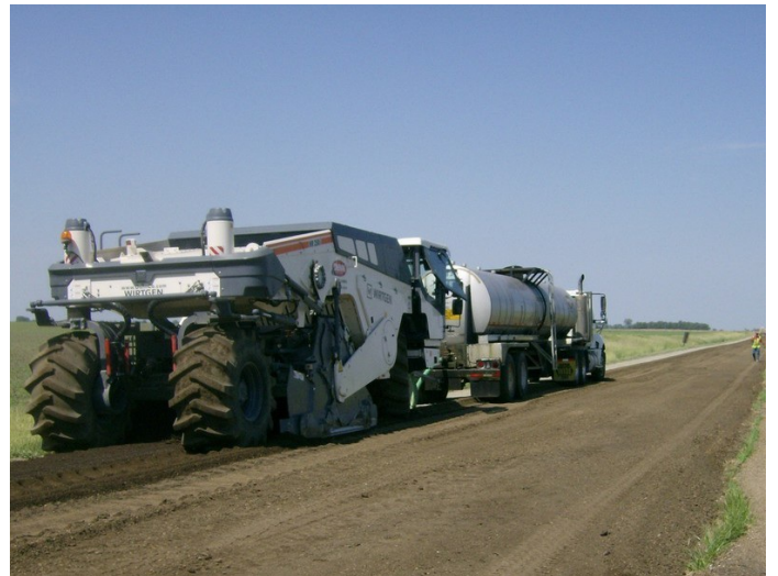
FDR Stabilization with Engineered Asphalt Emulsion
