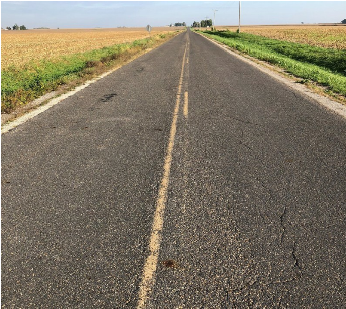
Original Narrow, Distressed Pavement
