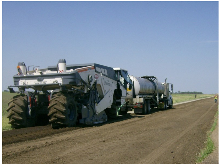
FDR Stabilization with Engineered Asphalt Emulsion
