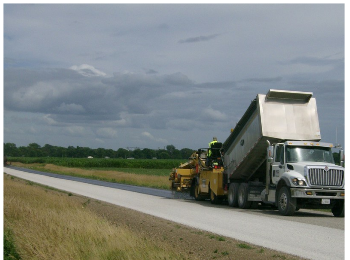
Part 1 of the Cape Seal was Chip Seal with HFP Emulsion
