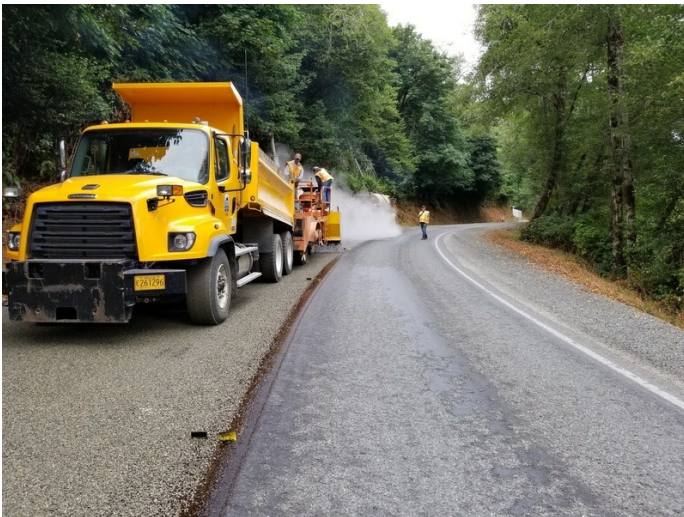
Chip seal in process
