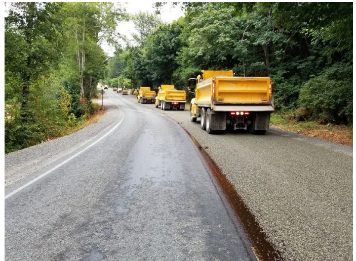
Chip seal in process
