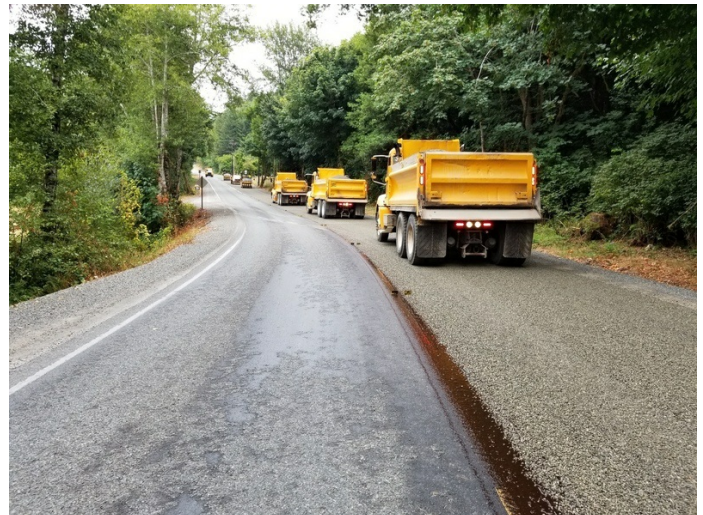
Chip seal in process
