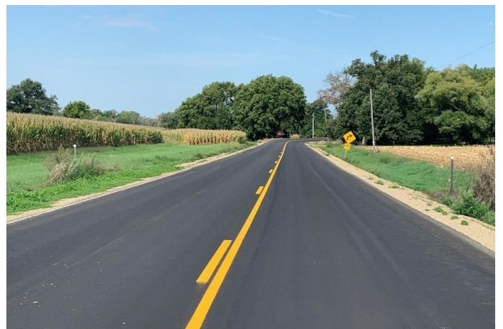
Finished Project with Cape Seal Surface
