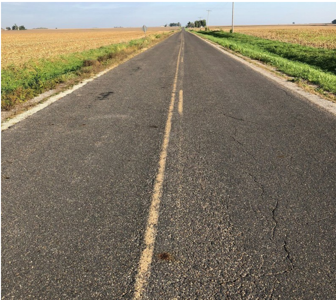
Original Narrow, Distressed Pavement
