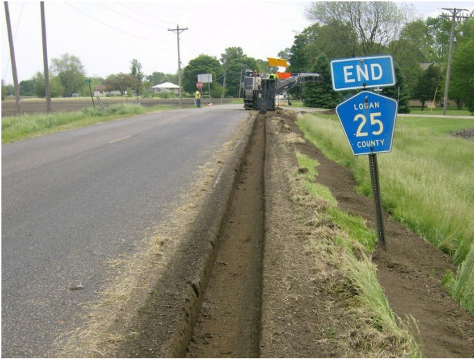
Trenching Material for Widening with FDR
