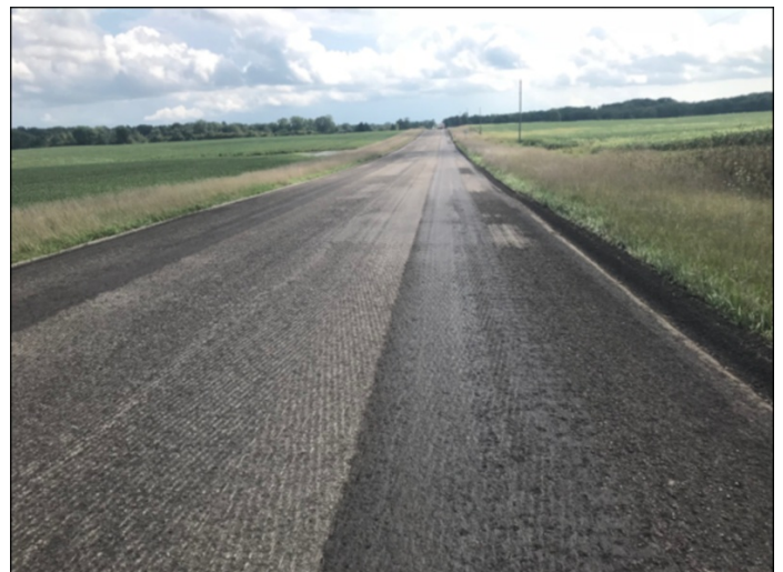
CCPR Mat after Profile Milling
