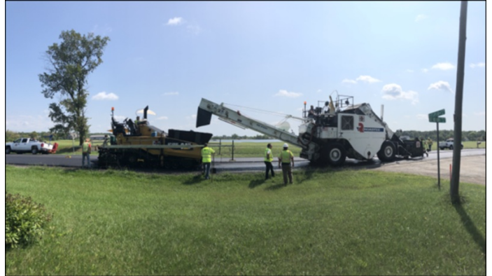
Paving of the 2.0-inch 12.5mm HMA surface
