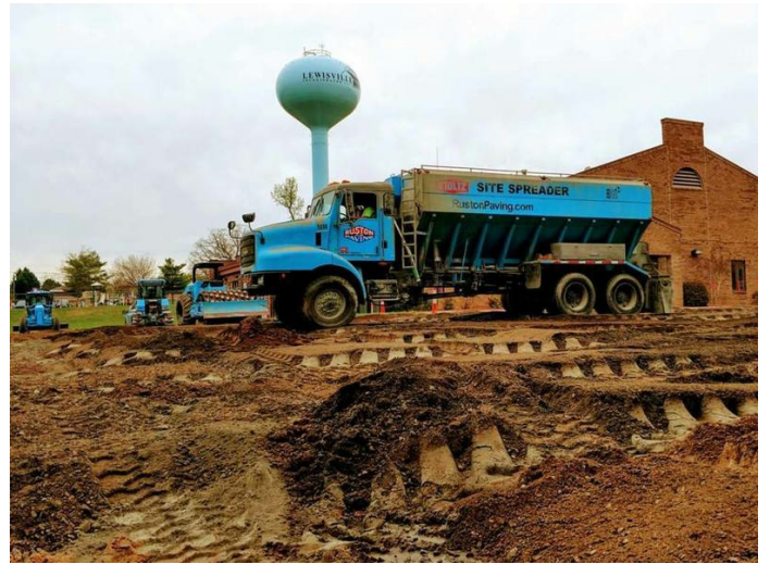
Applying and mixing Portland cement
