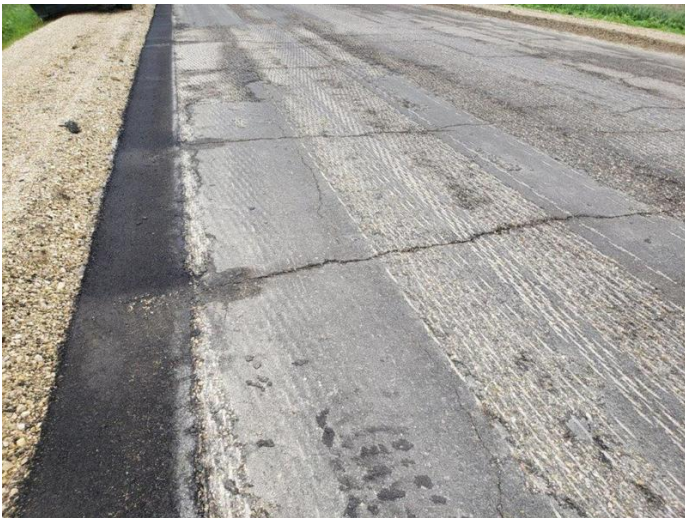
Sinclair Ave after profile milling
