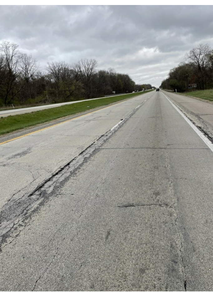
Existing Pavement Surface during Investigative Sampling
