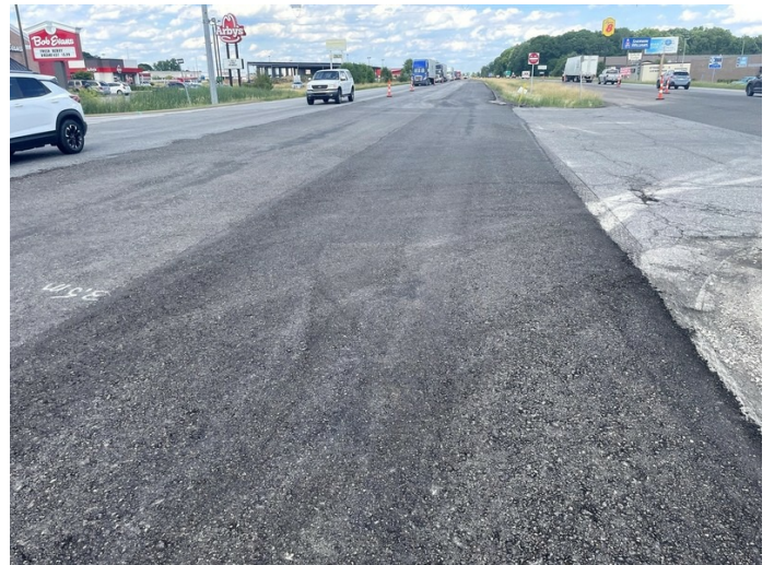
Due to heavy traffic volumes, the CIR mat was opened to intersection traffic directly after compaction with little to no raveling observed
