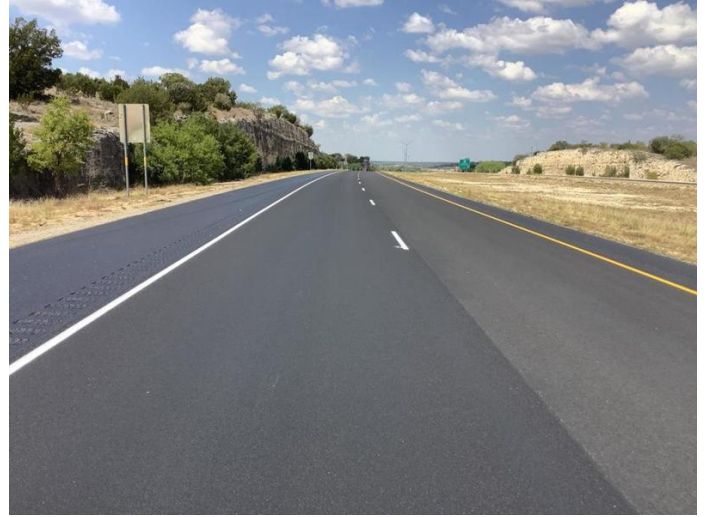
Completed Micro Surfacing project in Ozona, Texas maximized surface friction.
