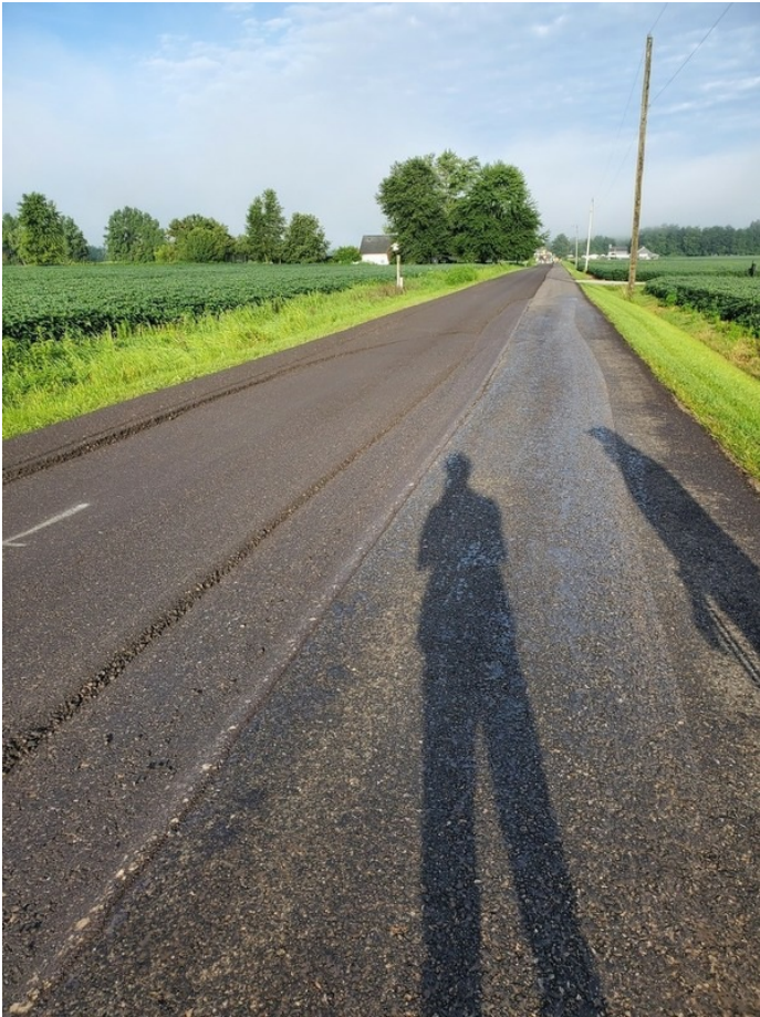
Compacted and uncompactd CIR mat on Jackson Road
