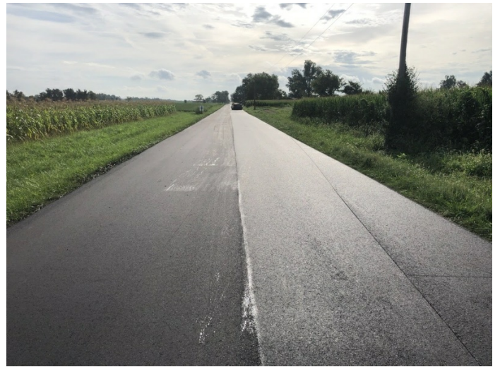
Finished 1.5-inch HMA surface on Jackson Road
